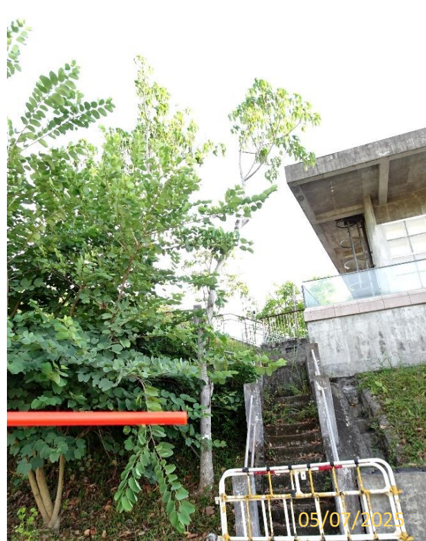
T113 – General View
