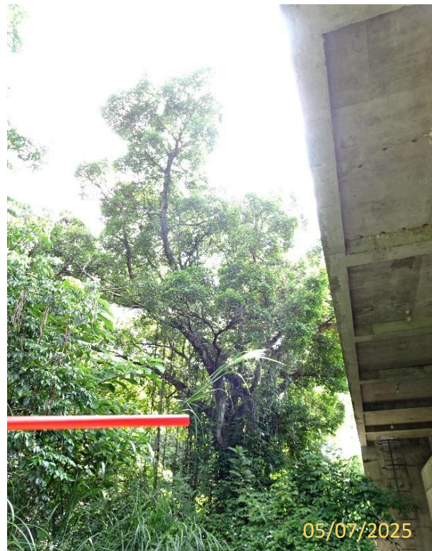
T135 – General View
